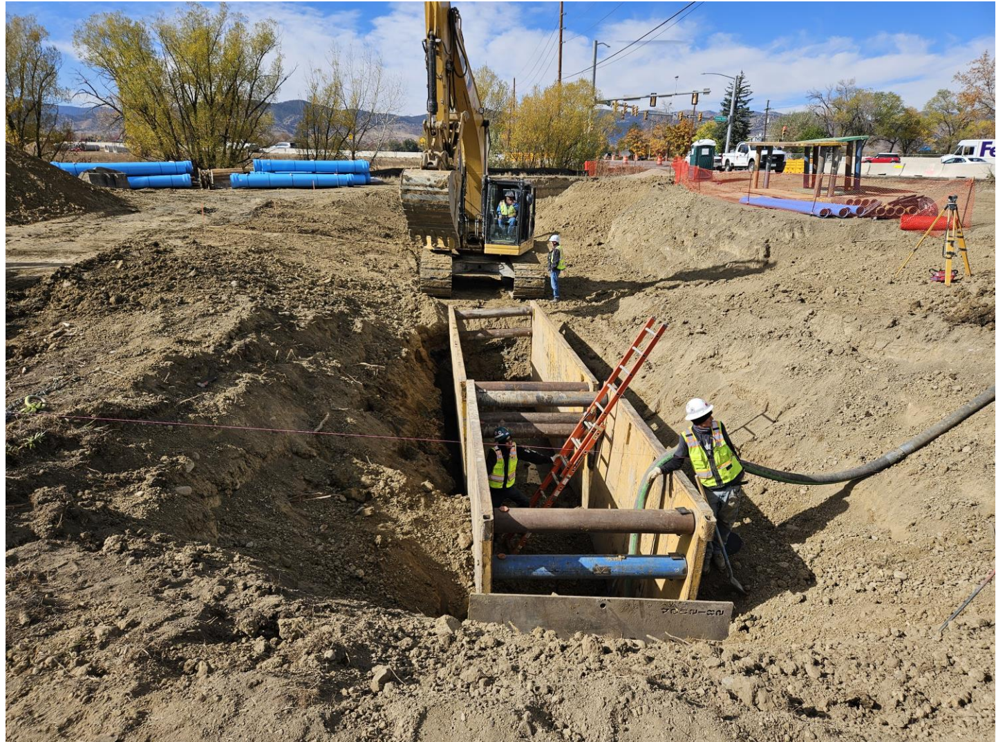
Jay Road Left Hand Water District Waterline relocation
